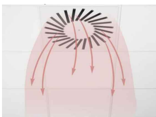
Vertical air discharge (heat air supply)
